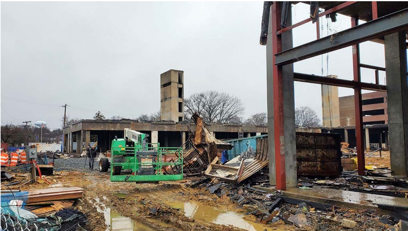
Remains of South Alex after the February 8 fire. Photo courtesy of Covering the Corridor
