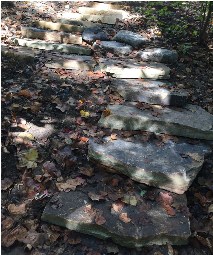
Steps range in height from 3.5 to 5.25 inches
