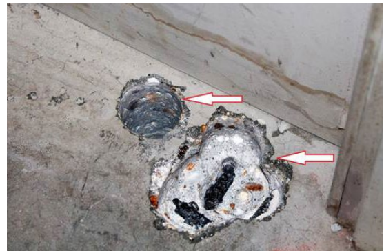
In another unit on a different floor, the drill team made multiple attempts to penetrate the core.
