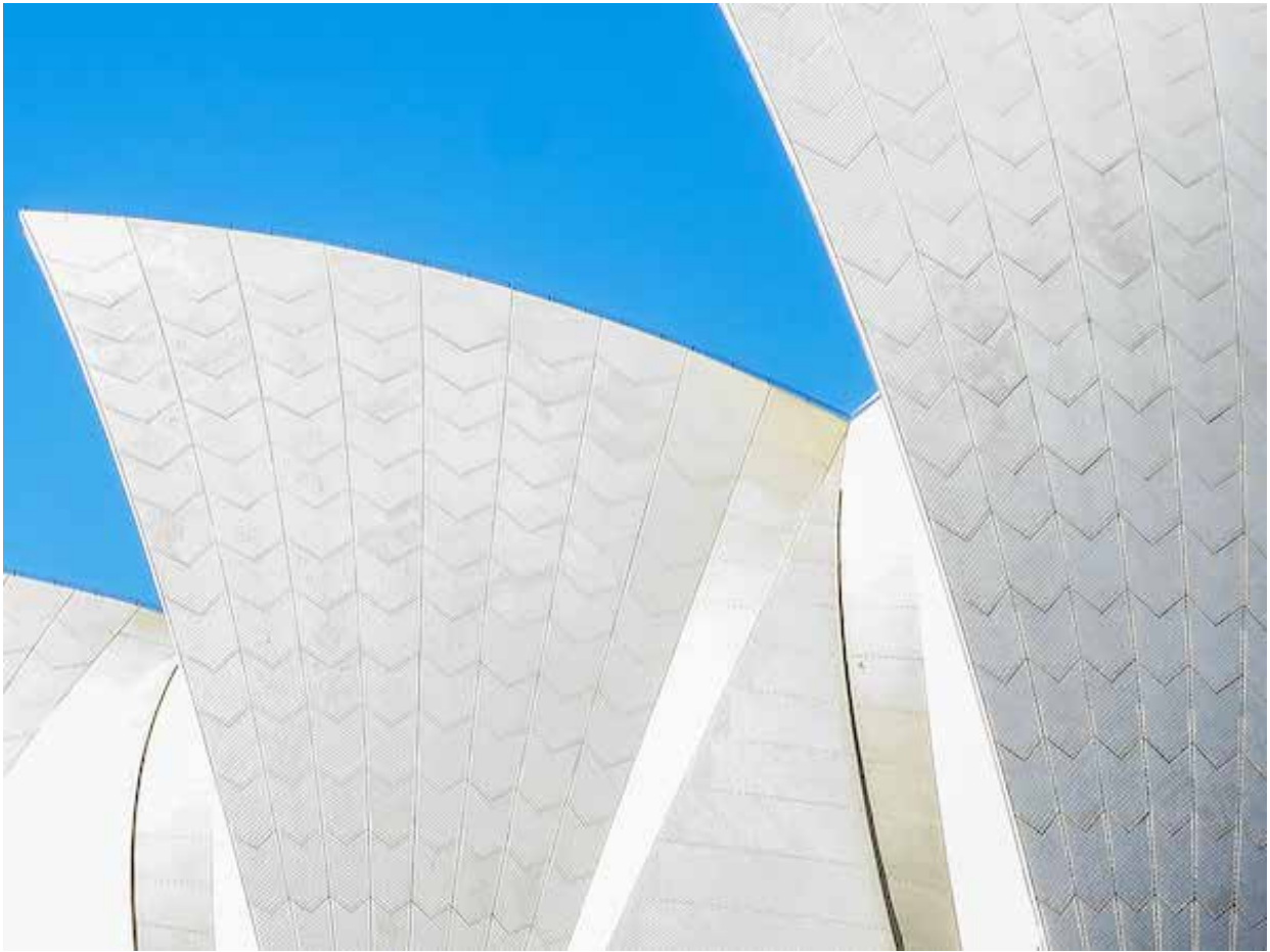
Sydney Opera House roof detail
