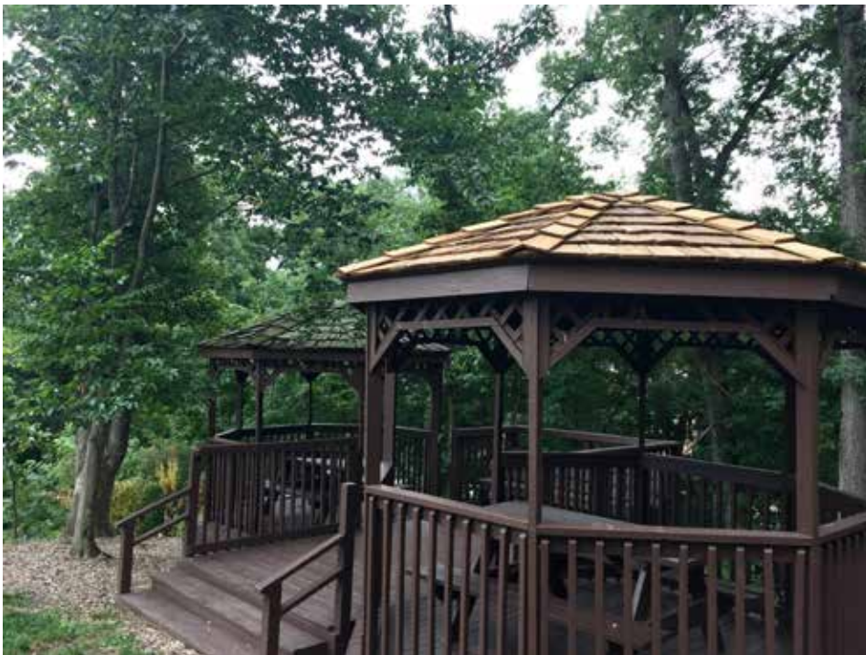
The gazebos are undergoing much-needed repairs to the roofs
