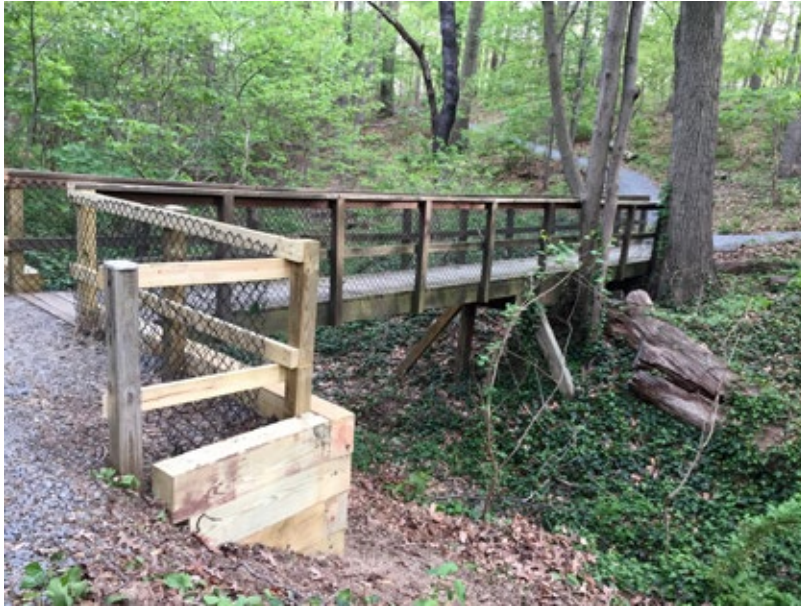
The bridge was reinforced with new wooden buttresses
