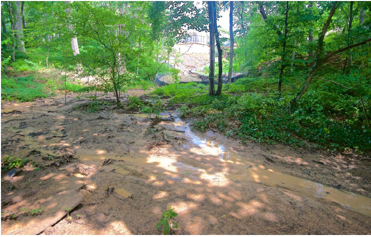
(Left) Erosion resulting from removal of trees.
