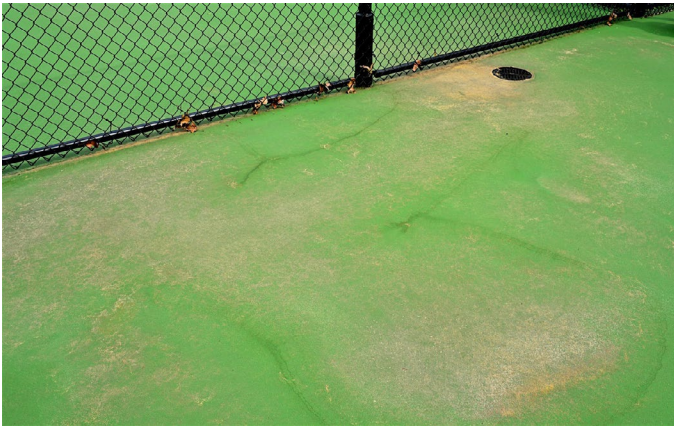
(Left) Poorly maintained first resurfacing. Was it known that this had to be replaced because of the poor construction?
